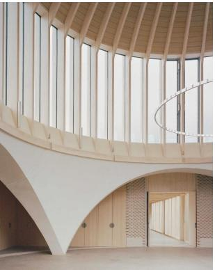
A 12m-diameter circle determines the inner temple, helping focus the congregation's attention onto a central altar. The space is enclosed by a pendentive structure supporting a lantern and dome, akin to those seen in Byzantine, Renaissance and Baroque churches, with arched openings to the cardinal points in the pendentive. Supporting a circular timber and glass lantern above, this structural element's form is modelled as a three-dimensional expression of the energy lines crossing the site.
