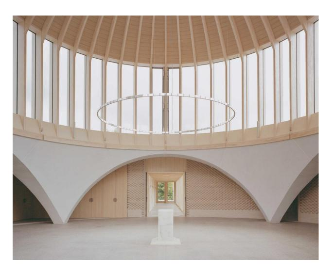
The acoustics within this space were also tricky, due to its composition from four different materials set at various angles. As such, the use of materials and treatments internally also became very technical: the use of textured brick to scatter sound and perforated ash (the pinholes so tiny they're only visible upclose) acting in place of acoustic baffling. The sound is surprisingly even from every part of the room.
