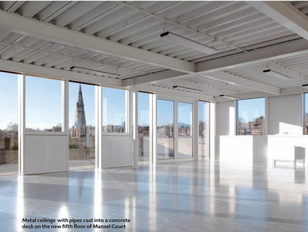
Metal ceilings with pipes cast into a concrete deck on the new fifth floor of Mansel Court
