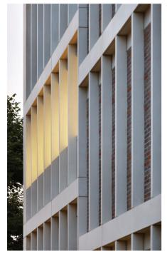
The deep window reveals help both to provide shading to the interior and reduce solar gain
