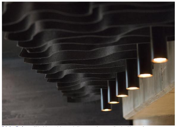
**Light fittings:** Working with specialist manufacturer Static, Haworth Tompkins conceived the foyer lighting as a single, conglomerate installation formed of 500 dimmable LED lamps encased in rolled copper mesh to diffuse and warm the light. Each individual light is made of two copper mesh sheets, bound by thick copper wire and suspended from high-level tracks.
